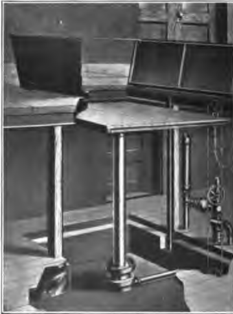
Fig. 106. Typical Plunger Hydraulic Sidewalk Elevator
